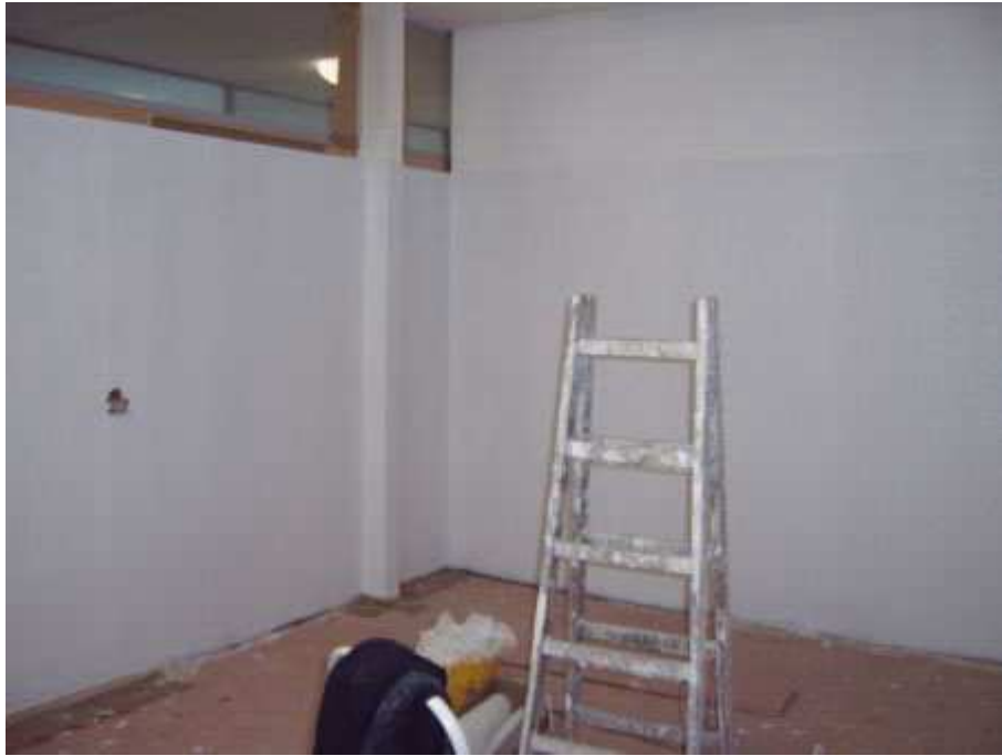
The surface of X-Shield is prepared with primer
