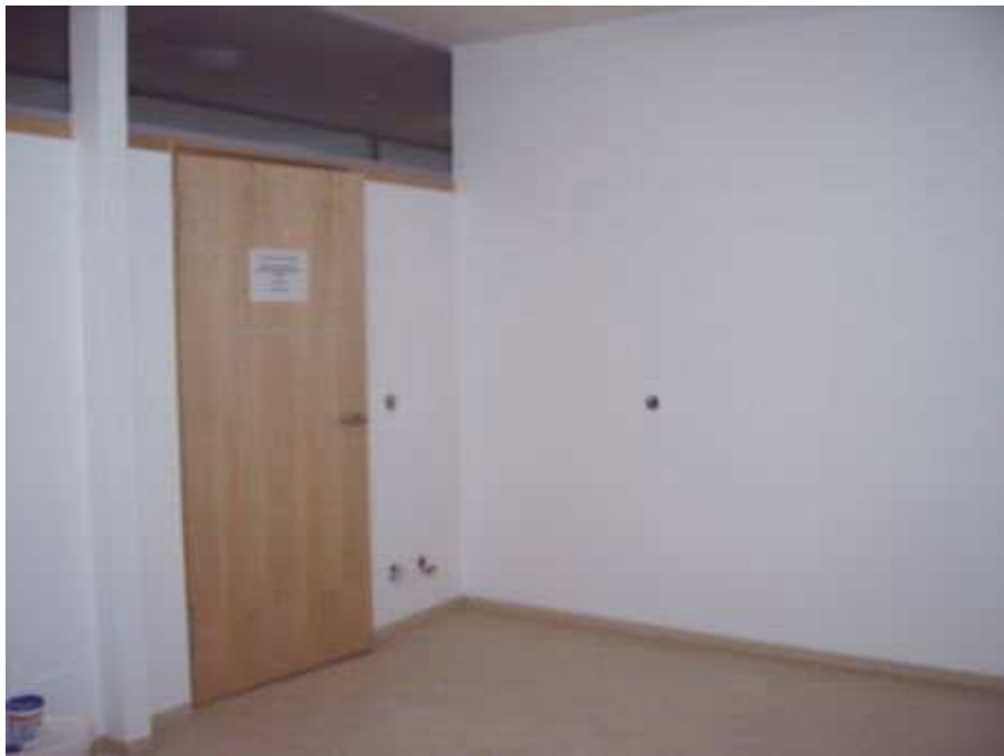
The new room for X-Ray use is ready.
