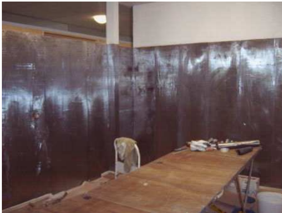
Installation of X-Shield
