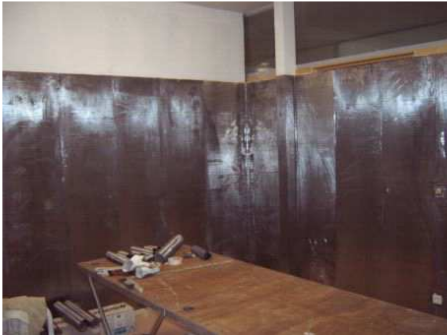
Installation of X-Shield
