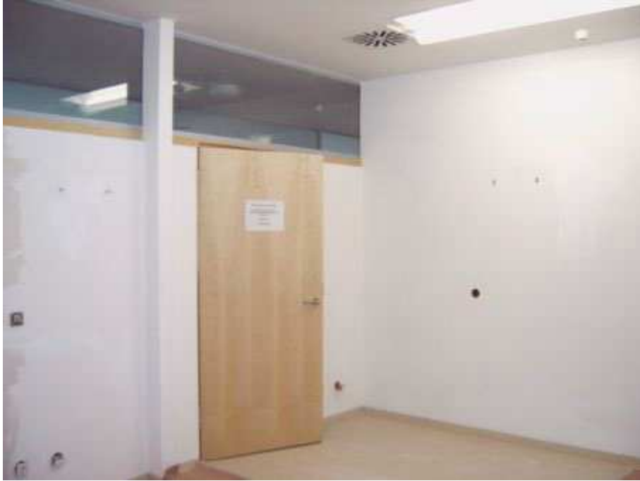
The fibreglas wallcovering is painted
